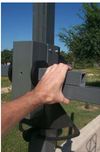
4. Manually rotate mounting arm 90 degrees counterclockwise.
